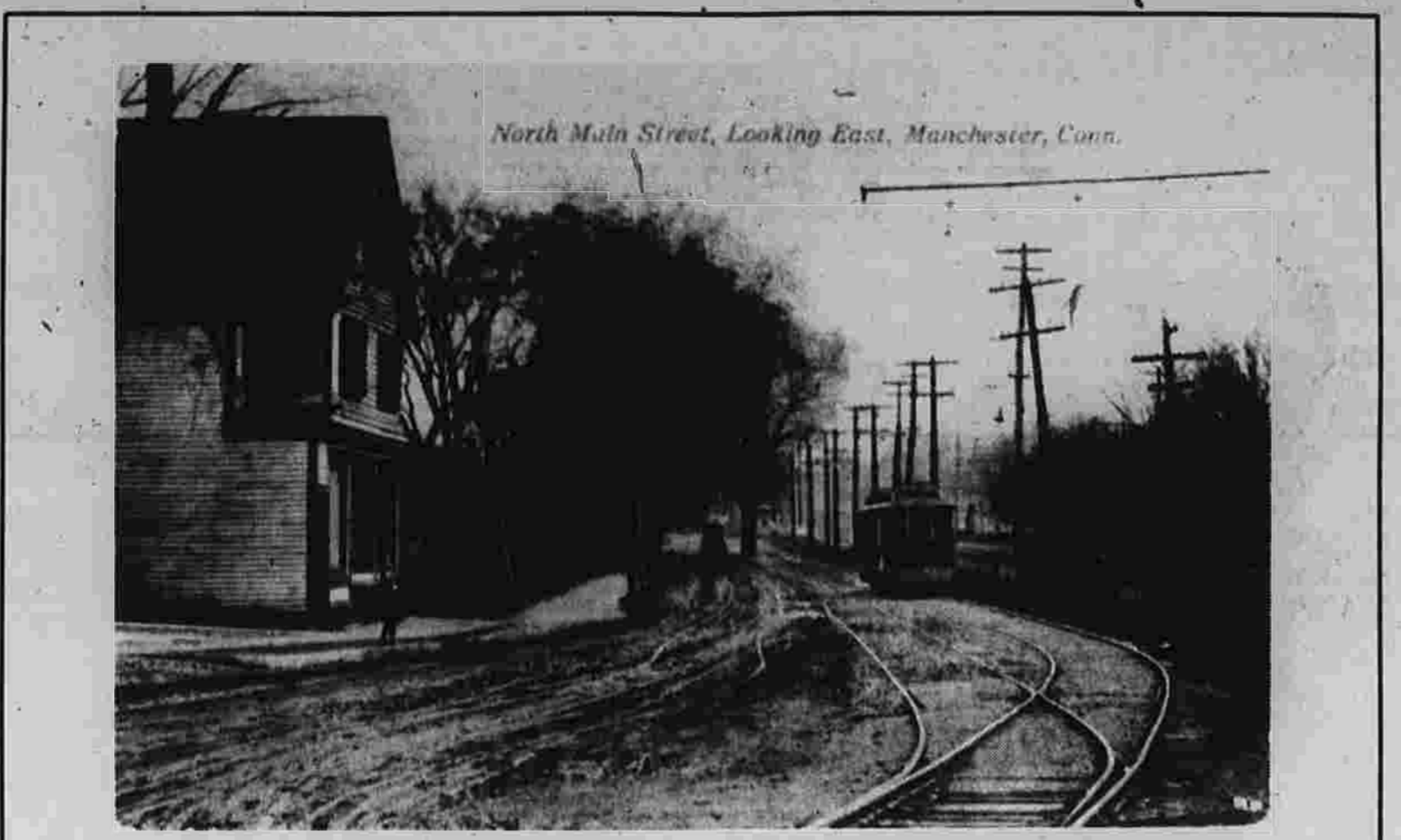
North Main St. in this view looking east, once ran closer to the railroad tracks than it does today. Double trolley tracks at this point provided running room for cars going to Hartford and to Rockville and Stafford Springs. (Courtesy Mrs. Marilyn Mann, 255 Summit St.)
